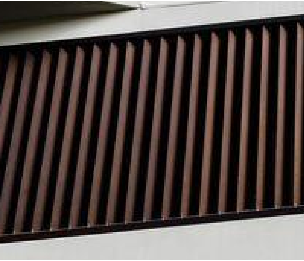
LV2 LOUVRES TYPE 2 VERTICAL ALUMINIUM BLADES
