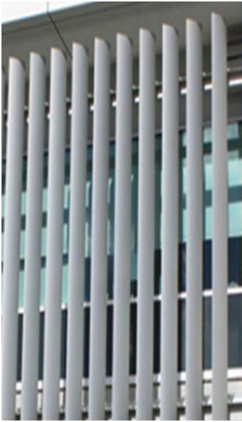
LV1 LOUVRES TYPE 1 VERTICAL ALUMINIUM BLADES
