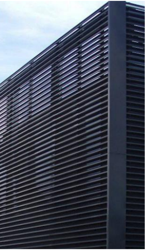
LV3 LOUVRES TYPE 3 DARK GREY HORIZONTAL WEATHERPROOF LOUVRES
